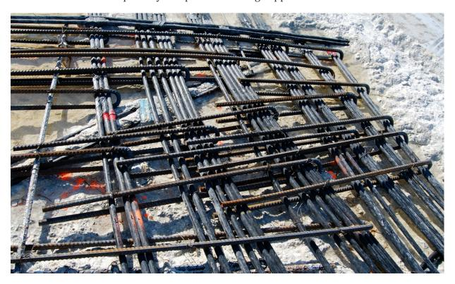
Photo: Supplemental hairpin reinforcement added at banded tendon lateral sweep repair.
