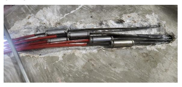
Photo: Installation of these splice couplers within the tendon sweep places an excentric load on the hardware.
