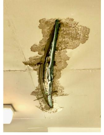
in the concrete, depending on the bending or shear moments at a particular point. This profile is readily accommodated within the concrete member and is rarely cause for concern unless there are large sections of concrete that need to be removed.
