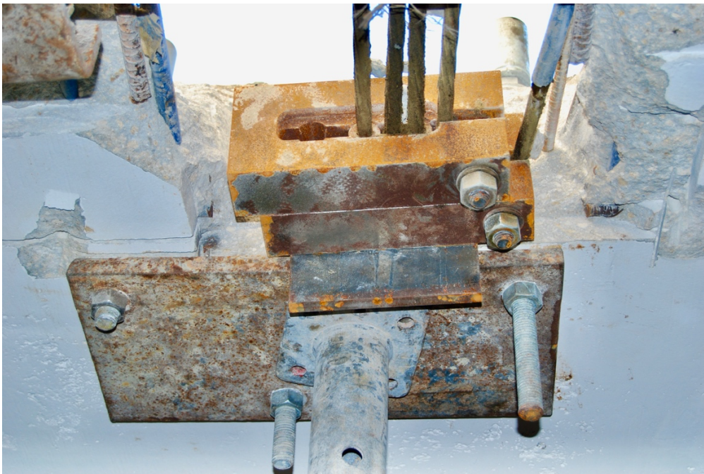
Photo: Field use of photo of the Patented Multi-Cable Lock-Off anchor used to secure bundled cables
