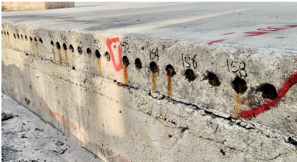
Image 6: Anchors placed too close to the surface and lacking adequate stressing anchor pocket coverage.
