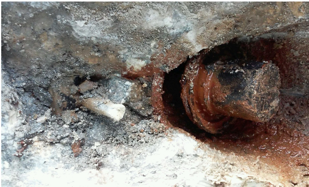
Image 8: Water leaking from anchor after pocket grout removed.
