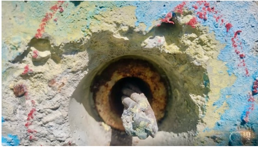
Image 3: Cable found with missing wedges after the grout was removed.
