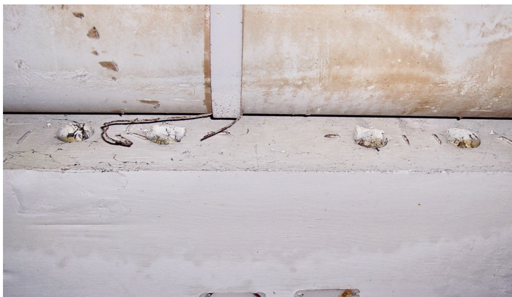
Image 7: Unfilled anchor pockets located at interior expansion joint.
